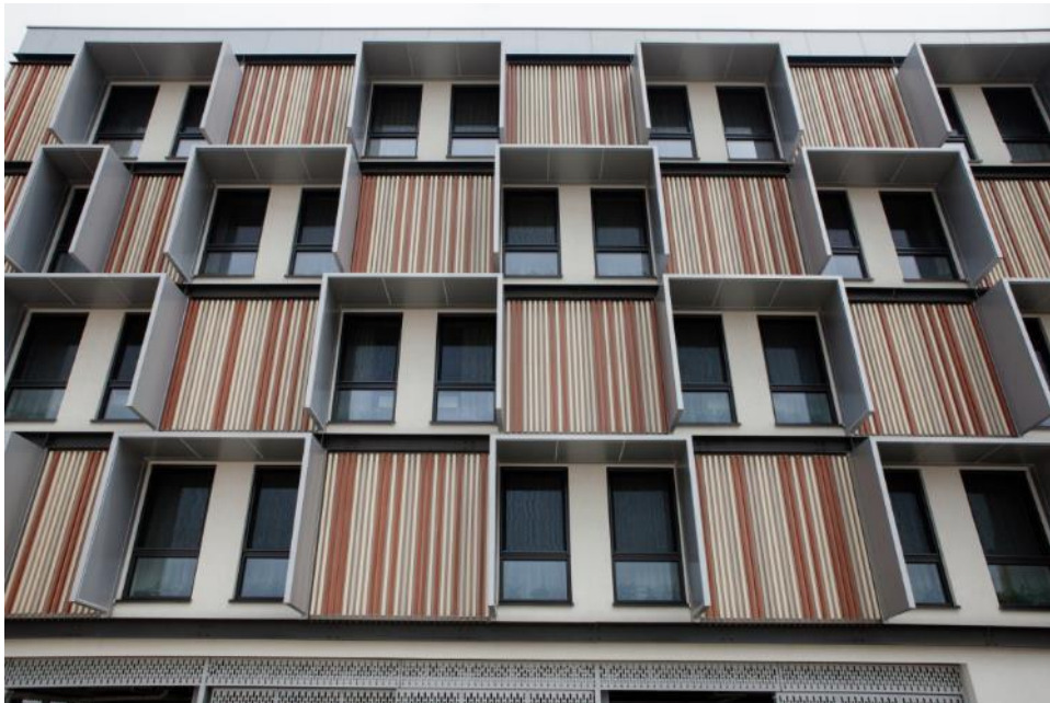
Figure 6: The passive house hotel, innovative neopor® insulation, efficient spray foam insulation for the roof (Source: BASF)
