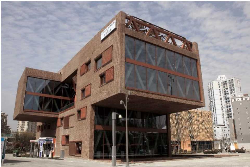
Figure 5: The hamburg house: thin and efficient insulation for the external walls and healthy indoor air (Source: BASF)
