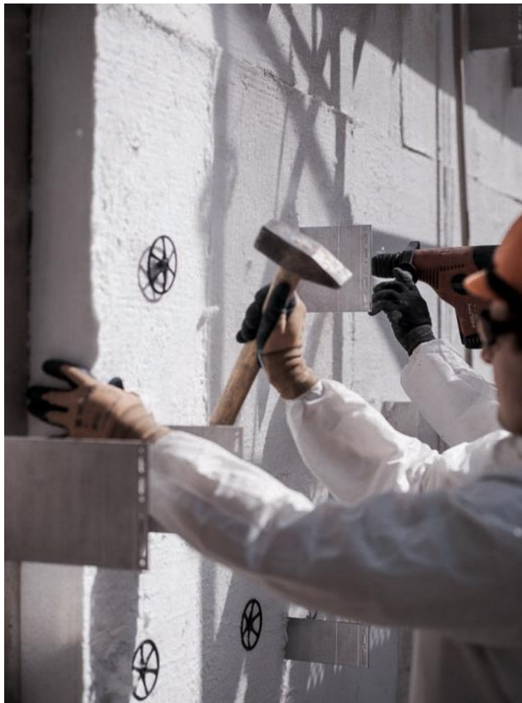
Figure 4: Aerogel insulation for space saving (Source: BASF)
