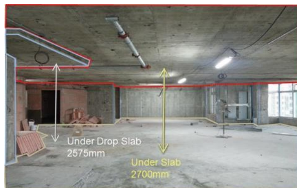
Figure 6: Existing structural ceiling level
