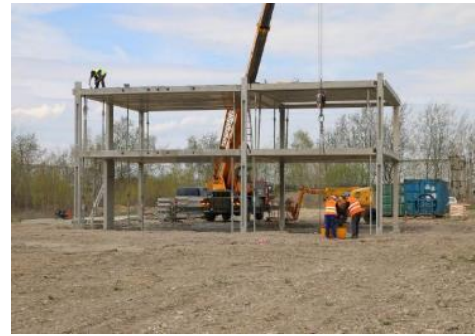
Figure 9: Finished load bearing structure of experimental OSEEB frame
