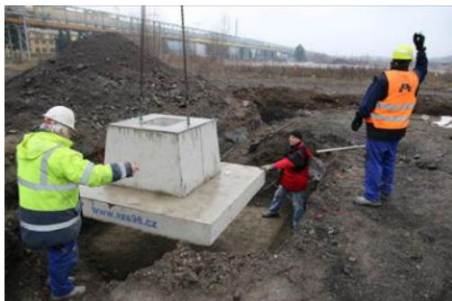
Figure 4: Precast pocket footing
