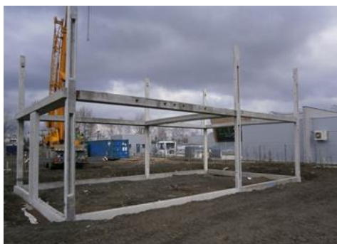
Figure 6: Structure of the 1 st floor
