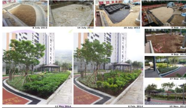
Figure 7: Construction of ZIS at trial planter
