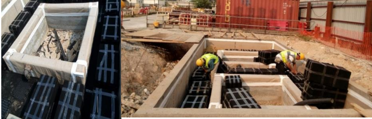
Figure 9: Construction of ZIS at trial planter at Homantin Site
