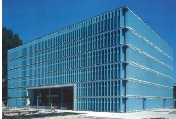
Figure 1: EMPA zero energy office
