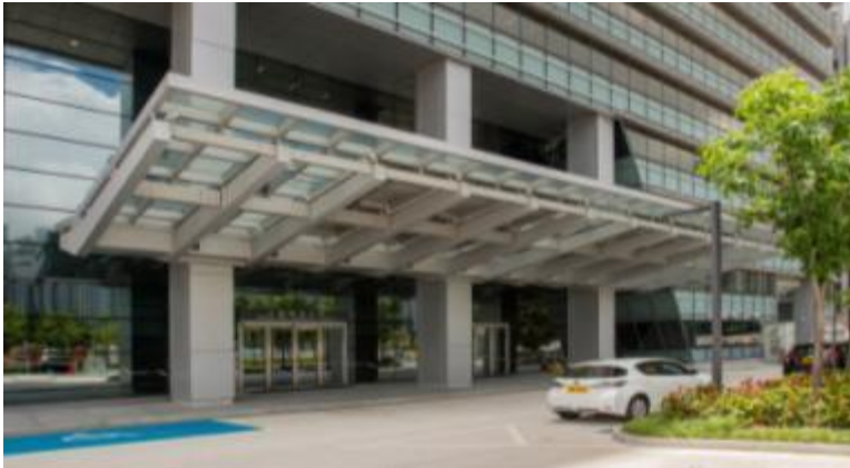
Building integrated photovoltaic panels in canopy
