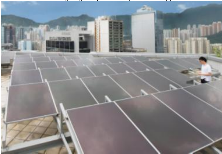
Photovoltaic panels on upper roof
