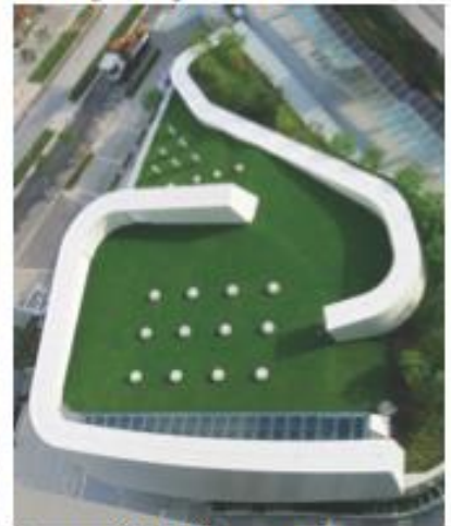
Community hall green roof
