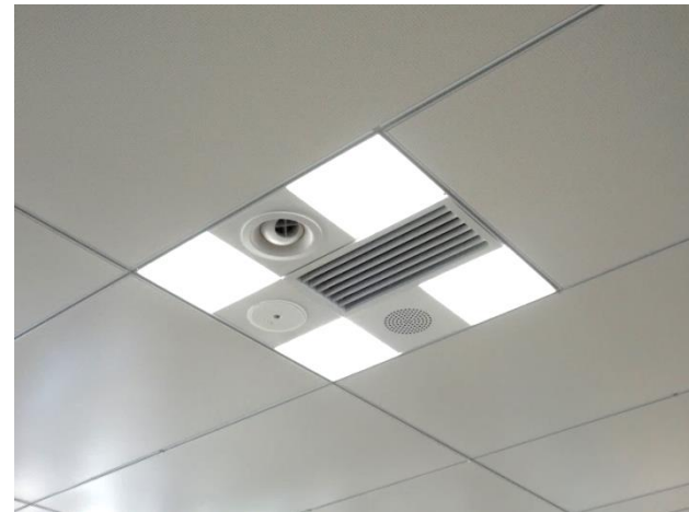
Ambient LED lighting 300Lx & Thermal human sensor
