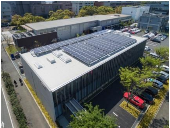
Devices on the roof
