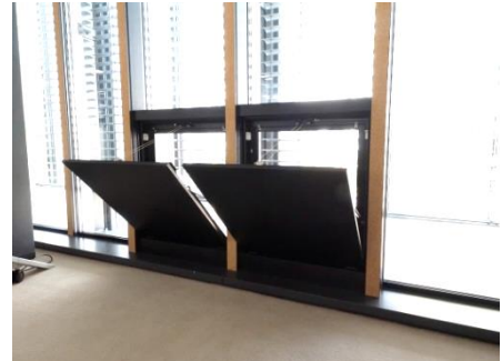
Natural ventilator (auto control)
