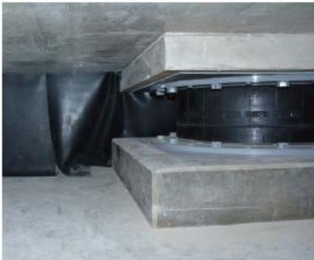
Seismic Isolation space for cool/heat trench
