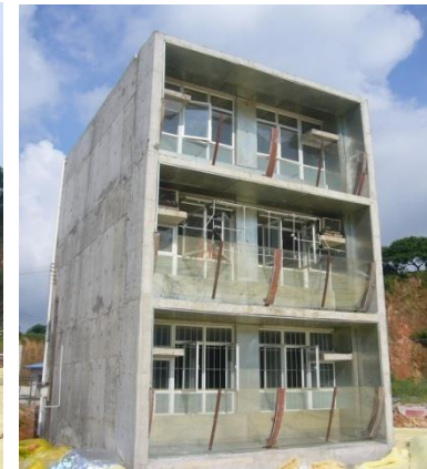
Scenario 6 – Polymethyl methacrylate (PMMA) parapet, ceiling & side walls with absorptive surface
