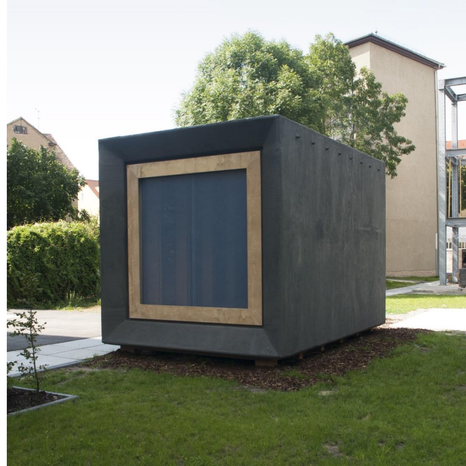
West elevation with window made of prestressed ETFE foil
