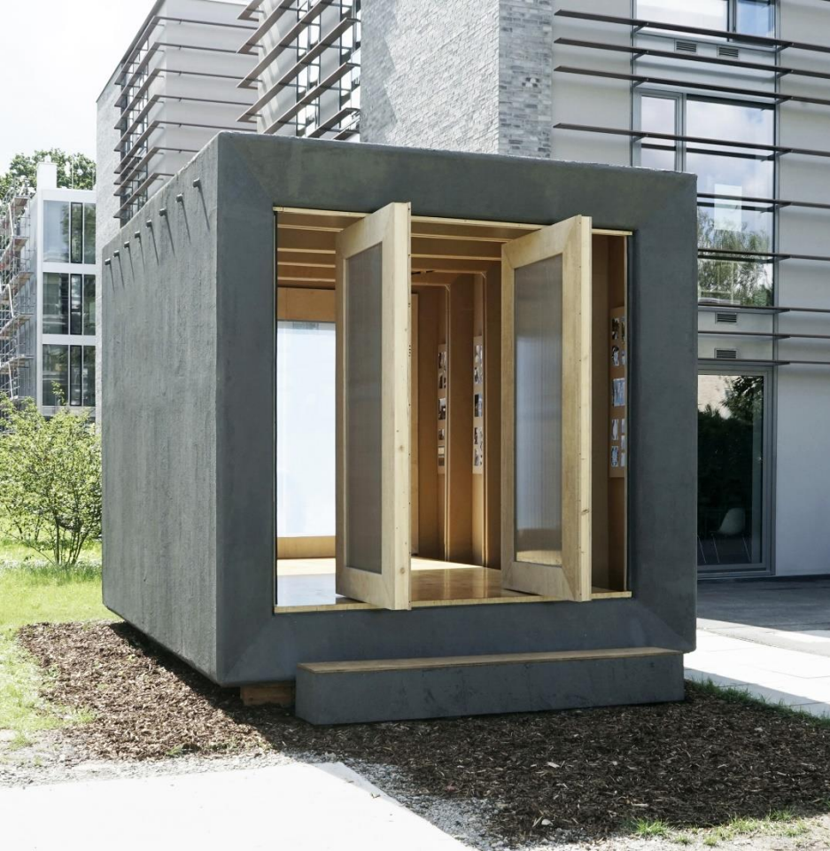
Finished building with two-component sealing on the facade
